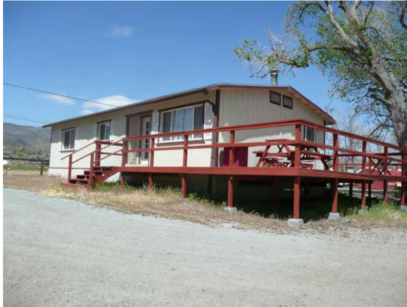
Modular Motel Units
