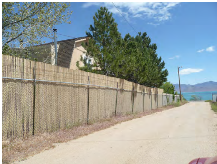
Figure 2-14 – Existing Permitted Screen Fence
