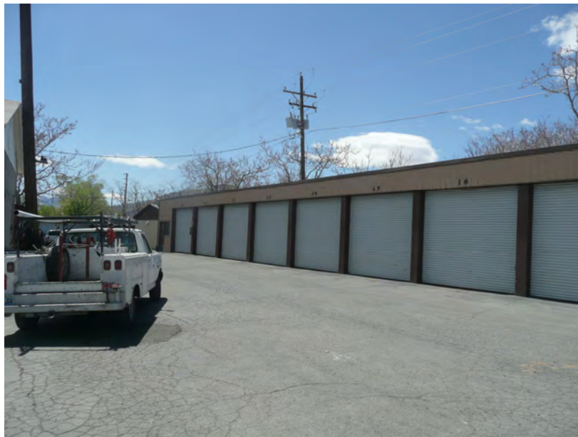
Enclosed Storage (located behind Lodge/Marine Shop)
