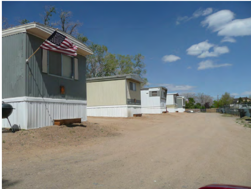
Modular Motel Units
