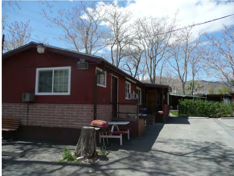
Motel Building (located south of Lodge building)
