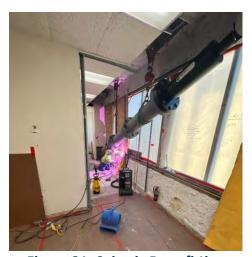
Figure 31: Seismic Retrofitting in the City of Reno City Hall
