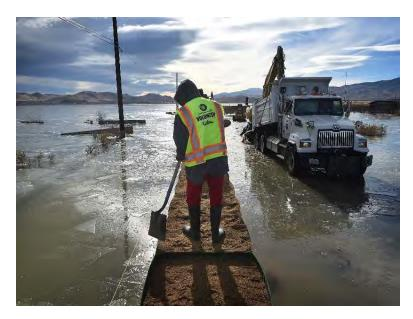
Figure 97: Flood Barriers Being Set Up on the Edge of Swan Lake by Washoe County<sup>170</sup>
