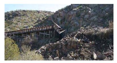
Figure 45: Water Flume Damaged by the Mogul-Somersett Earthquake, 2008<sup>98</sup>
