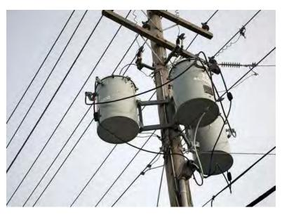
Figure 74: Utility Pole with Power Lines and Transformers<sup>121</sup>
