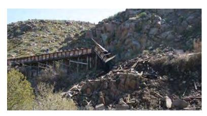
Figure 82: Water Flume Damaged by the 2008 Mogul–Somersett Earthquake<sup>222</sup>
