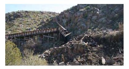
Figure 11: Water Flume Damaged by the 2008 Mogul-Somersett Earthquake<sup>40</sup>
