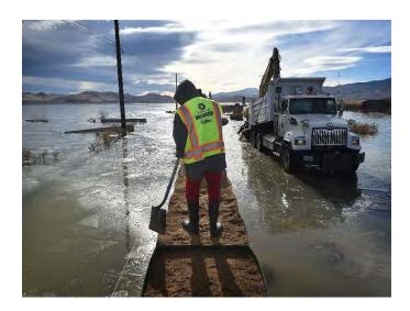
Figure 18: Flood Barriers Being Set Up on the Edge of Swan Lake by Washoe County<sup>49</sup>
