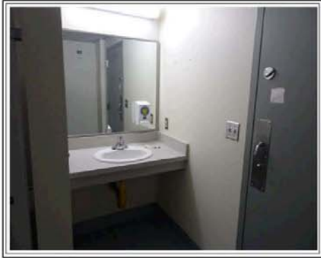
WOMEN'S RESTROOM IN THE BASEMENT
