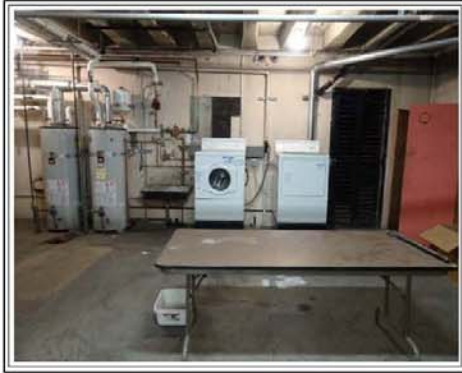
MECHANICAL/STORAGE/LAUNDRY ROOM IN THE BASEMENT
