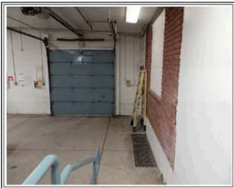
GARAGE AREA LOCATED AT THE REAR OF THE FIRST FLOOR
