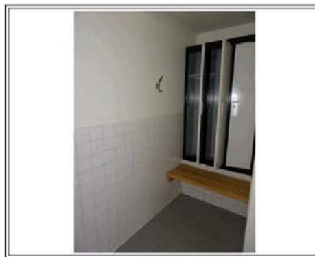
MEN'S RESTROOM IN THE BASEMENT
