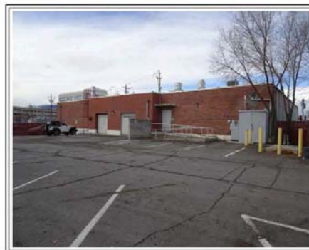
EAST (REAR) SIDE OF THE SUBJECT BUILDING
