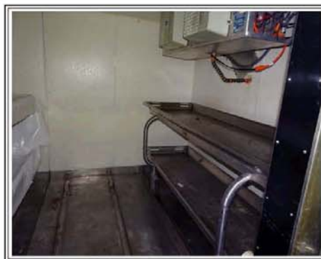
INTERIOR OF THE COOLER IN THE COLD ROOM IN THE BASEMENT
