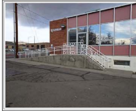
VIEW OF NORTHERN ENTRANCE INTO THE SUBJECT BUILDING
