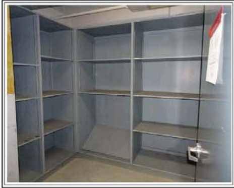
STORAGE ROOM IN THE BASEMENT
