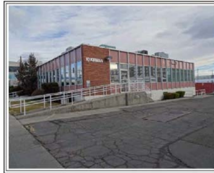
SOUTH SIDE OF THE SUBJECT BUILDING
