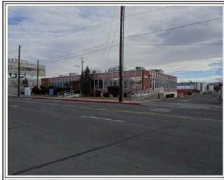
WEST AND SOUTH SIDES OF THE SUBJECT BUILDING
