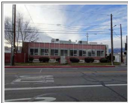
NORTH SIDE OF THE SUBJECT BUILDING
