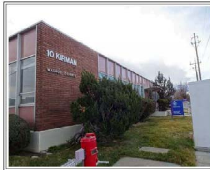
WEST SIDE OF THE SUBJECT BUILDING
