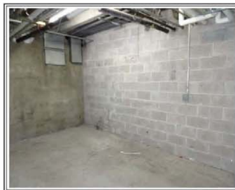
STORAGE ROOM IN THE BASEMENT
