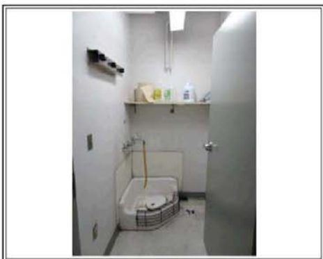
JANITOR'S CLOSET WITH WORK SINK IN THE BASEMENT
