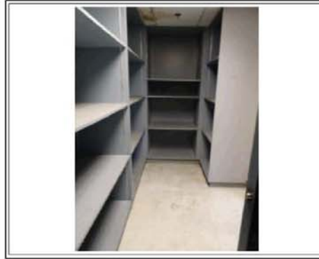
STORAGE ROOM IN THE BASEMENT
