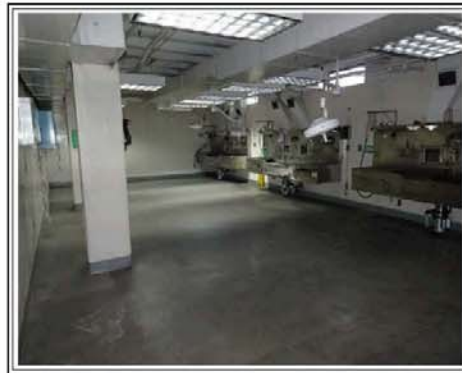
AUTOPSY ROOM IN THE BASEMENT
