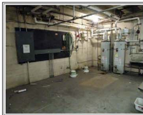
MECHANICAL/STORAGE/LAUNDRY ROOM IN THE BASEMENT
