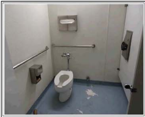
WOMEN'S RESTROOM IN THE BASEMENT
