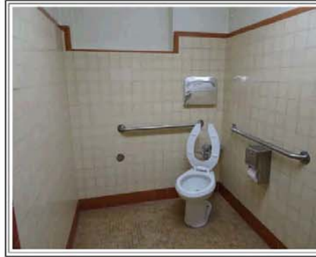
SINGLE USER RESTROOM LOCATED ON THE FIRST FLOOR
