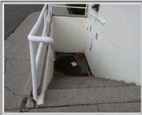
VIEW OF THE NORTHERN ENTRANCE INTO THE SUBJECT BASEMENT
