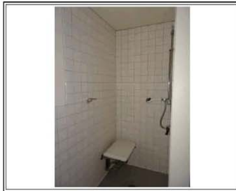
WOMEN'S RESTROOM IN THE BASEMENT
