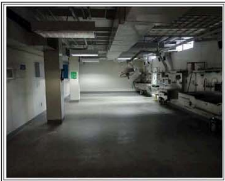
AUTOPSY ROOM IN THE BASEMENT
