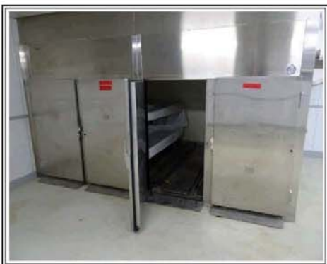
COOLER IN THE COLD ROOM IN THE BASEMENT
