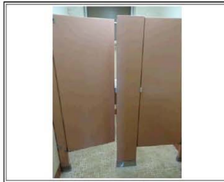
WOMEN'S RESTROOM ON THE FIRST FLOOR
