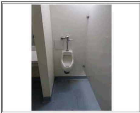
MEN'S RESTROOM IN THE BASEMENT
