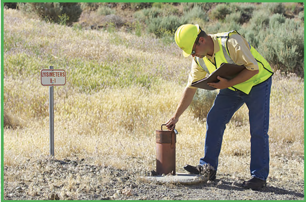
Figure 12: A technician checks a gas well at Lockwood landfill. (WM photo)
