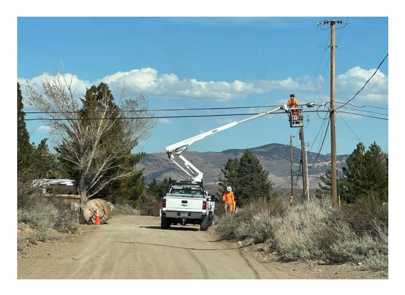
Same photo as on previous slide with width (~7') of truck duplicated to demonstrate size and space needed to properly service utility lines
