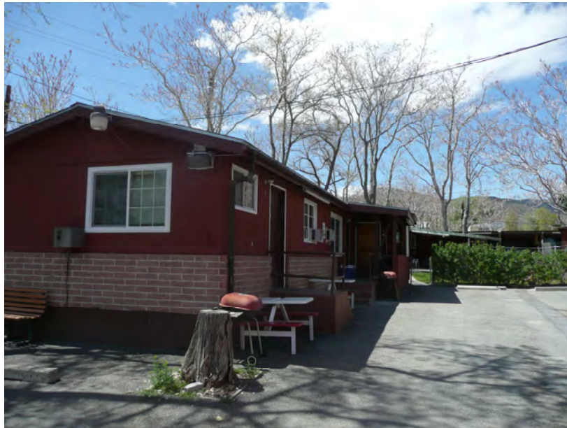
Motel Building (located south of Lodge building)
