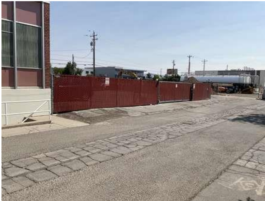
Subject Gated Entry to Fenced Area
