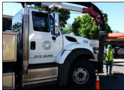
Jet Truck Operator, pulling the Electro Scan probe through the pipe, while surrounding it with water.
