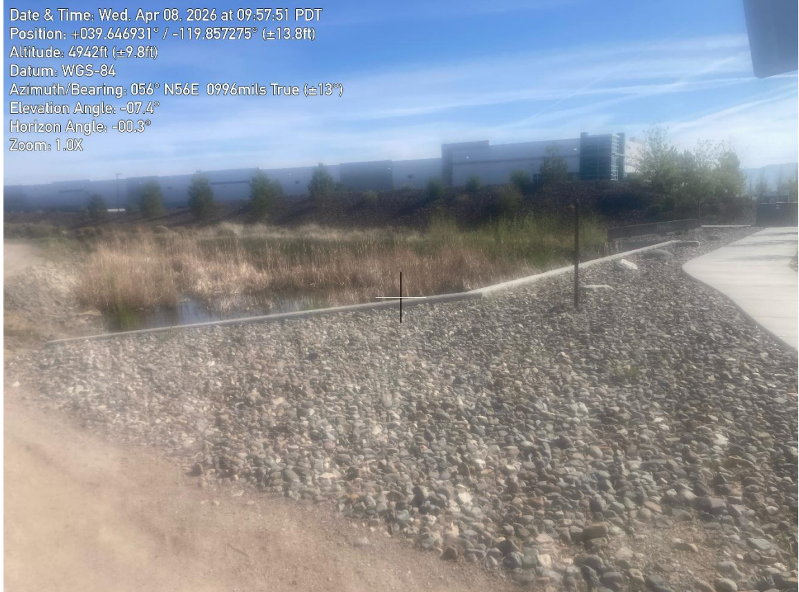
Photograph 12: Canal adjacent to the access road and the adjacent property to the east.
