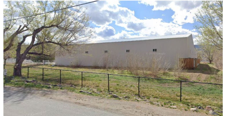
45 car garage at 1725 Holcomb Ranch Ln
