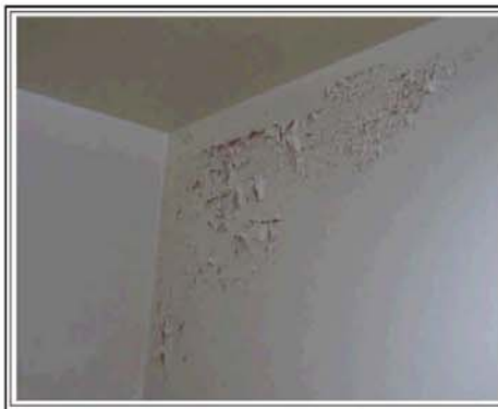
EXAMPLE OF WATER DAMAGE IN THE WALL OF THE UNISEX RESTROOM ON THE FIRST FLOOR
