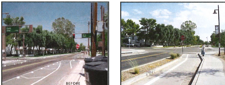
Photo 19: Examples of Addition of Transit Lanes without Removing Existing Auto Lanes
