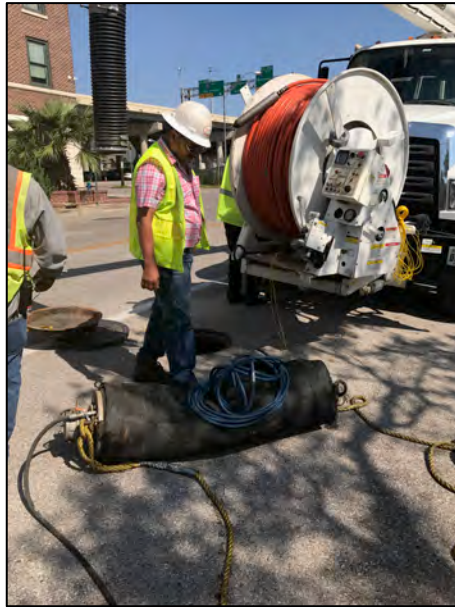
Plug inserted in 24" CIPP lined sewer mains in the City of Houston to surcharge pipe for 360-degree Electro Scanning Testing of pipe wall.
