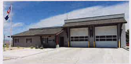
Station 36 - Arrowcreek 13500 Thomas Creek Rd., Reno
