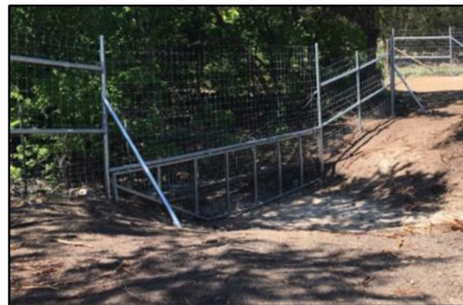
Photo 4 – Swinging Water Gate Example
