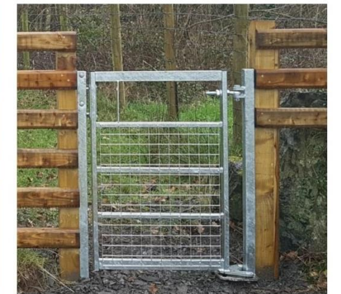
36 New Self Closing Pedestrian Gate
