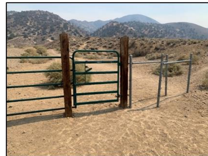
Photo 5 – Human Gap Gate and Small Manually Operated Panel Gate Examples
